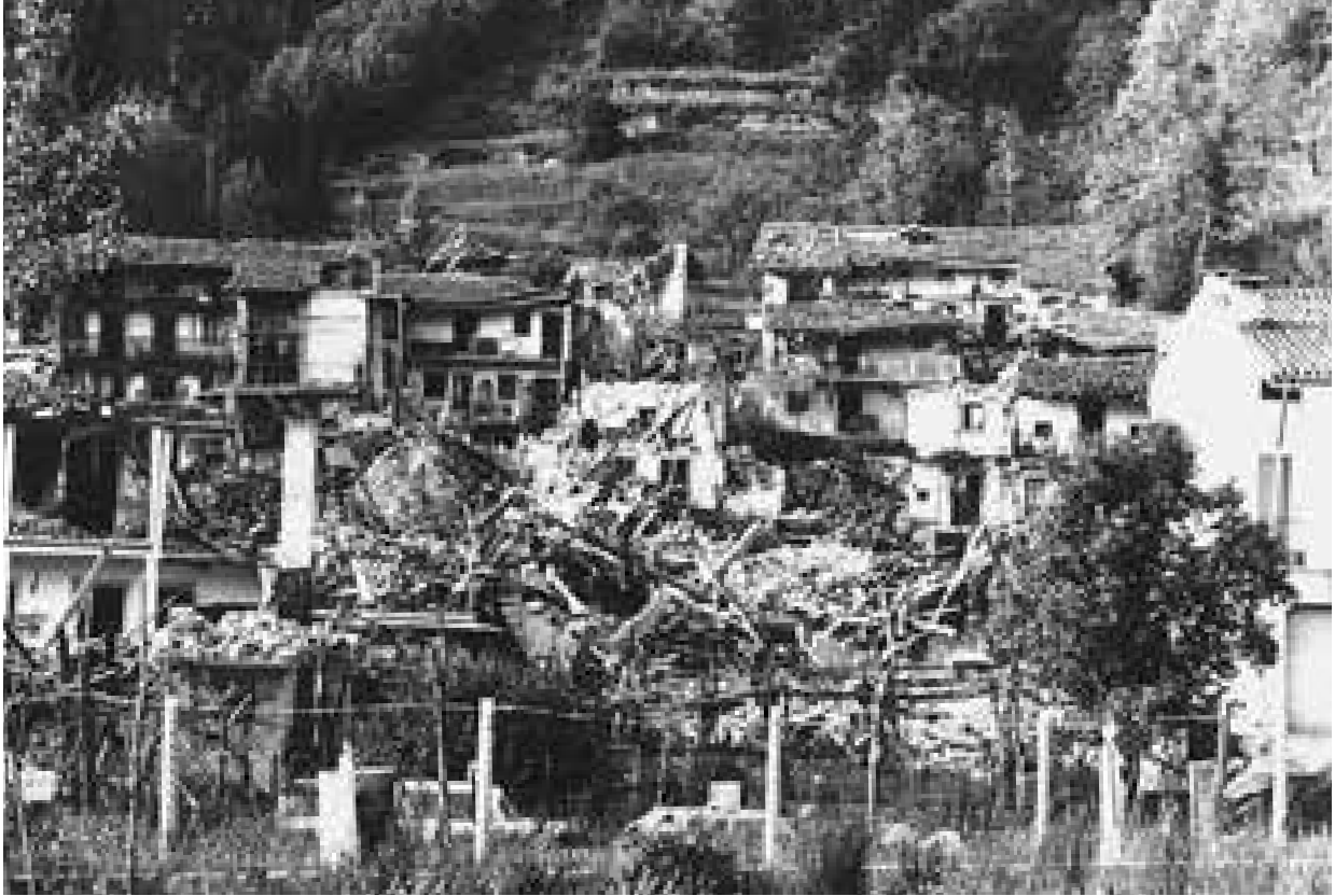
MONTENARS. Borgo Curminie
